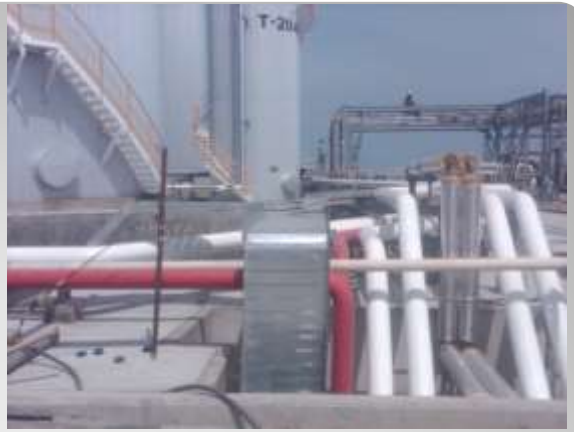
Product Name : Instal.Cable & Lighting Customer : PT Baria Bulk Terminal Location : Pulomerak - Cilegon.Banten
