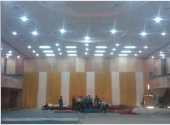
Product Name : Electrical Works Customer : STIKES Faletahan Location : Serang – Jawa Barat
