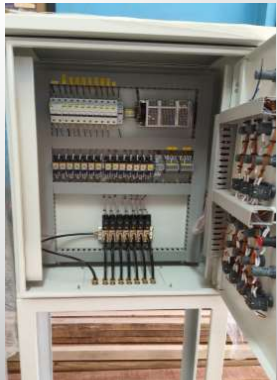
Panel MCC dan Panel Pneumatic Valve. PT.Coca Cola Customer : PT. AMRITA ENVIRO ENERGIA. Location : Pasuruan
