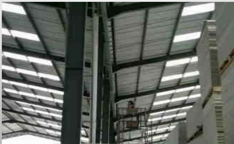
Product Name : Inst.Cable & Lighting Customer : PT. Bangunperkasa Adhitama Centra Location : Karawang
