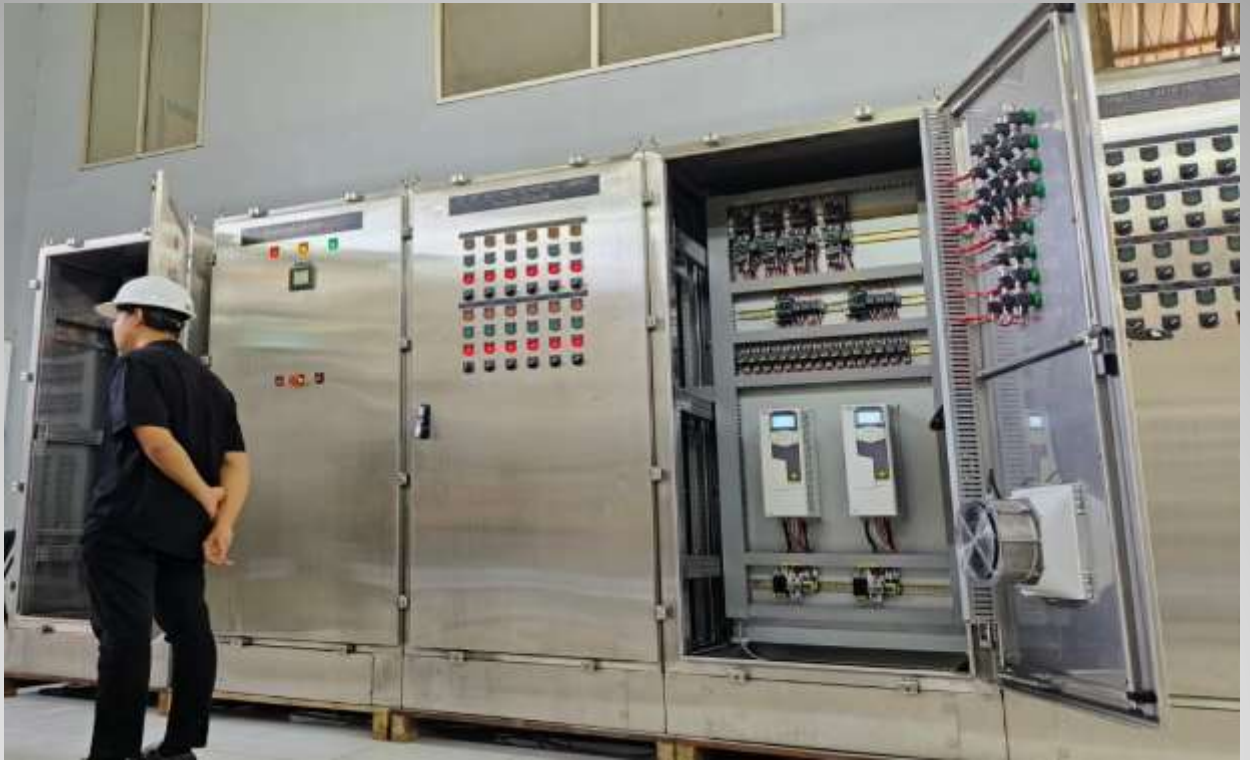
Panel WTP MCC dan Panel PLC di PT Amman Mineral Customer : PT. Amrita Enviro Energy Location : Sumbawa
