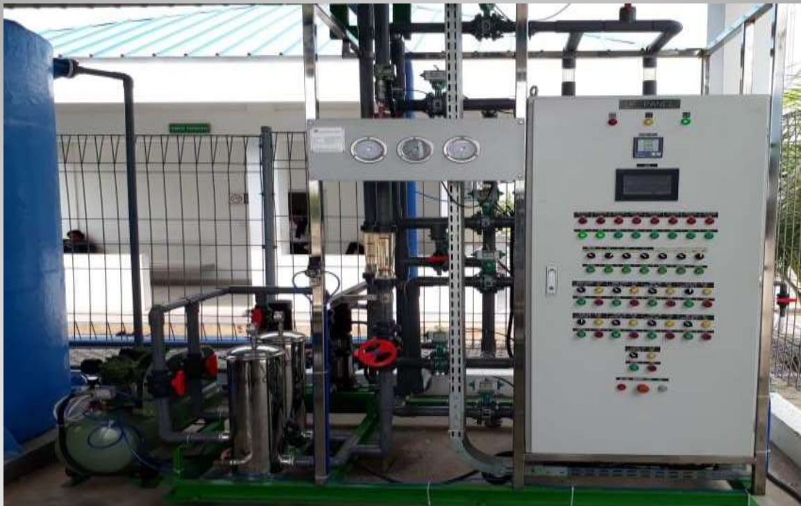
Panel UF at PT Indofood - Cirebon Customer : PT. Tirtakreasi Amrita
